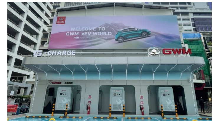
GWM fast charging station
